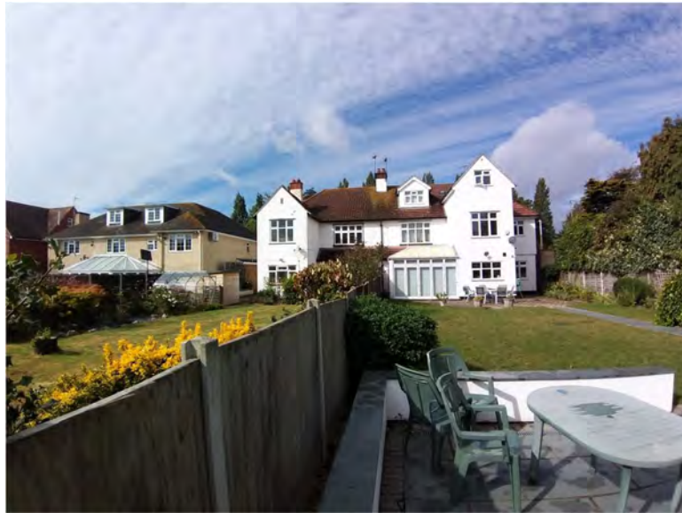
The site (right) and the neighbouring properties to the south.
